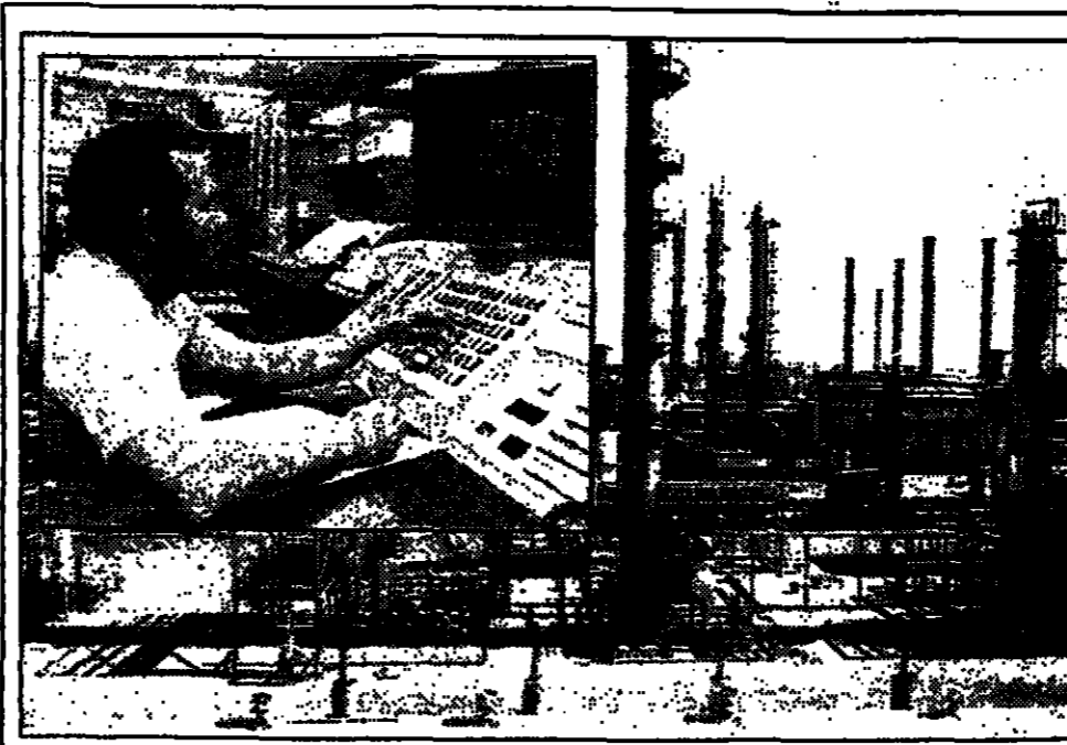
An oil refinery in Venezuela and its control room, which is computerized.
